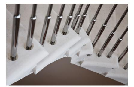
This contemporary home with its helical concrete staircase and mirror polished surroundings deserved a simple but elegant balustrade. CANAL produced individual mirror polished stainless steel spindle rods that were staggered to follow the line of the staircase. The rods were secured into the concrete at different intervals to ensure the symmetry and flow of the staircase through the home. To complete the sense of opulence, the balustrade was topped with a dark brown leather handrail.
